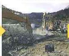
ソイルセメント攪拌混合 Churning and mixing of soil cement
