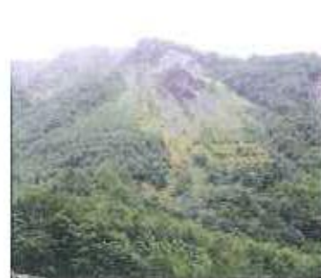
緑化後の斜面 Slopes after greening
