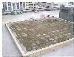
人工土壌の敷き均し Laying artificial soil
