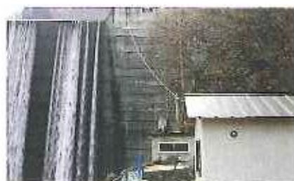
小水力発電の一例・堤防砂防えん堤 (長野県長野市) ダム堤高 25.0m 堤長 70.0m Example for Small Size Hydraulic Water Power Generation・Asakari Sabo Embankment (in Nagano city, NAGANO Pref.) Embankment spec Height: 25.0/Length: /70.0m
