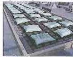
人工土壌の搬入 Carrying artificial soil
