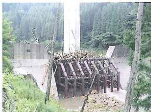
鋼製砂防えん堤 Steel sabo Dam
