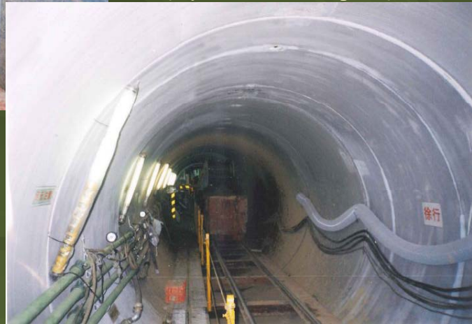
Muck transportation (by muck wagon)
