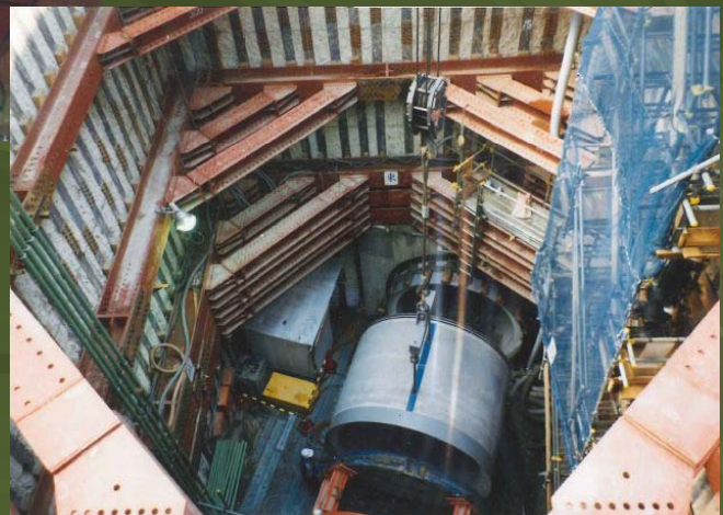
Launch of microtunnelling
