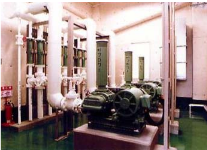
Blower used for blowing air into a contact oxidation tank
