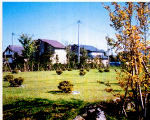
Ordinary scene. The water treatment system has been operating for 21 years under the grass.
