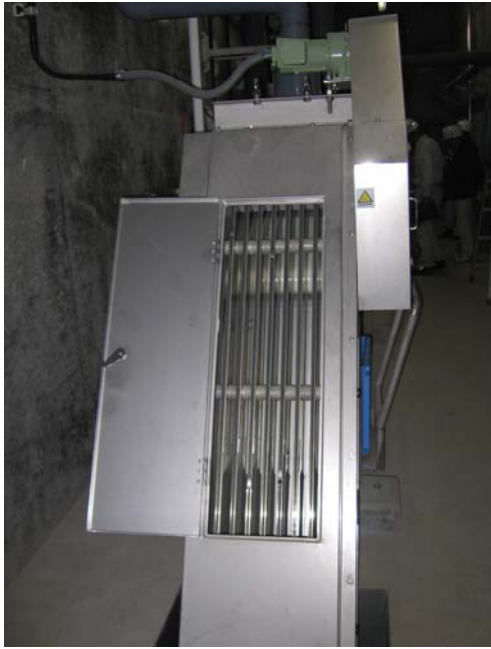
Coarse mesh screen with openings of 30 mm used in the Dojo-Joka System
