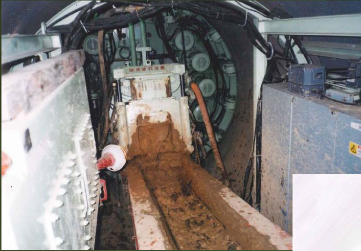
Muck discharge (behind the shield)
