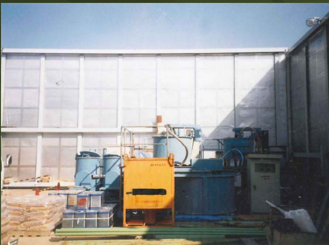
Lubrication & Backfill grouting Plant
