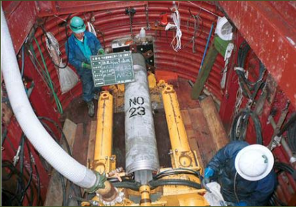
Liner plate sheeting
