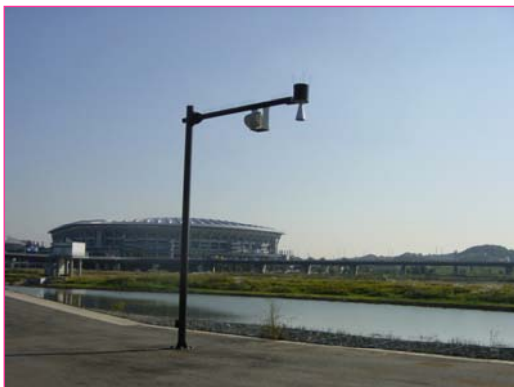
Overflow levee in retarding basin
