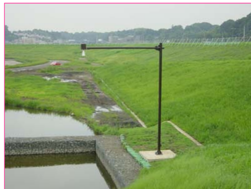
Reservoir Pond in retarding basin
