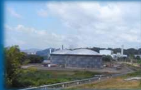
Fuel Pipeline and Tank Farm
