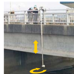
P C 桁の点検
