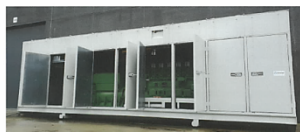
Container housing 1MW medium speed genset
